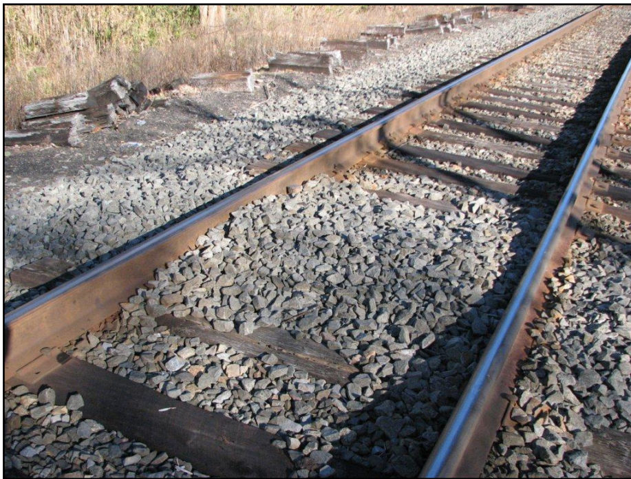
Figure 21: Modification to railroad track gravel bed to facilitate turtle crossing (photo courtesy of M. Musnick)
