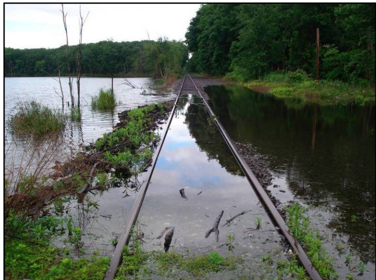
Figure 13: Haines Pond overflowing railroad tracks
